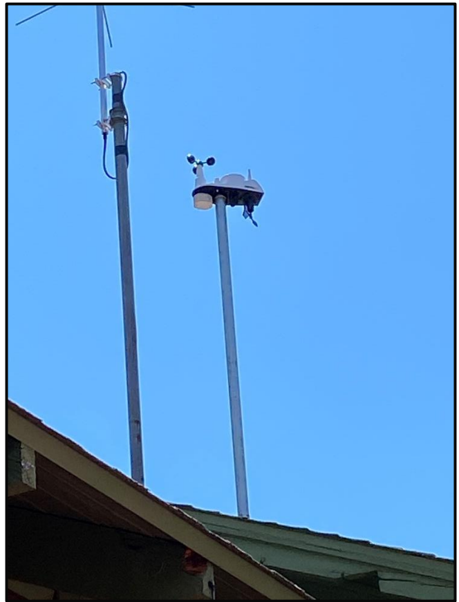
Weather Station at District Administration Office
