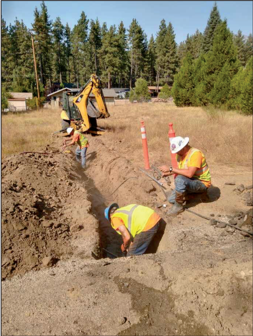
IWD crews installing pipe October 2020
