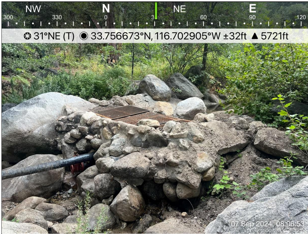
Photo 3. View of the water diversion structure.
