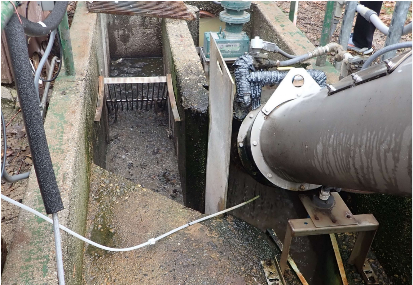
Figure 3: Existing Headworks Bypass Channel And Bar Screen
